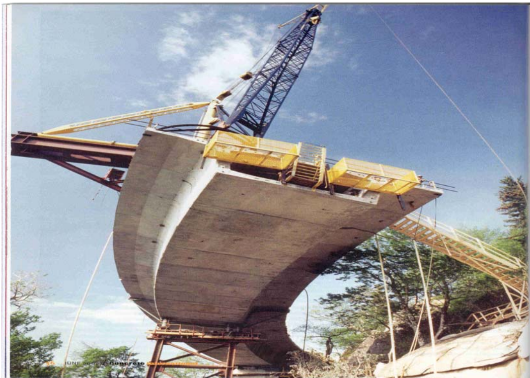
Figure B2. Construction of a Segmental Bridge
