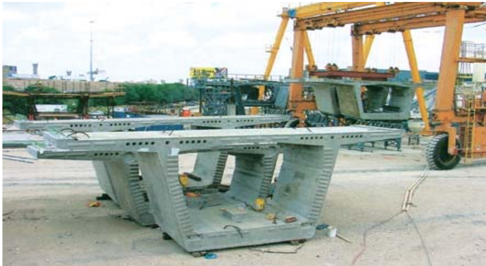
Figure B3. Segmental Components (Post-Tensioning Ducts Visible)
