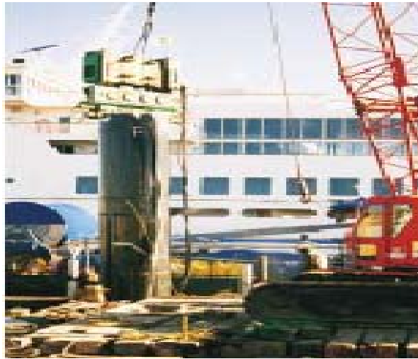
Figure A33. Installation of a Composite Monopile at Cape May, New Jersey
