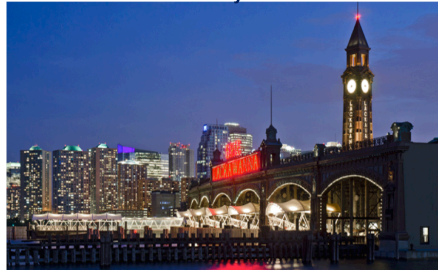
Hoboken Ferry Terminal
