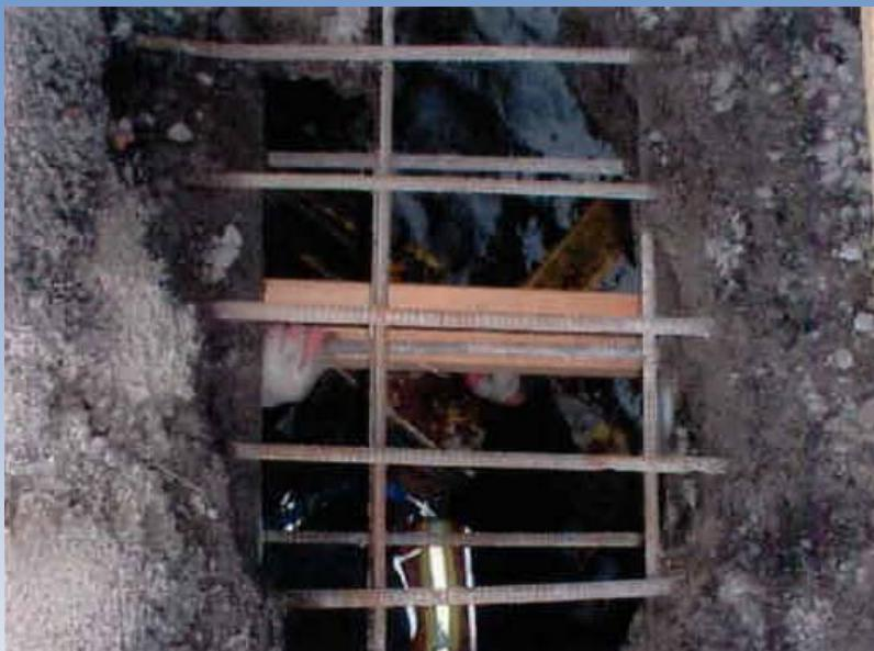
Collapse of closure pour in 2003 created hazardous conditions for motorists and required \$50,000 in emergency repairs.
