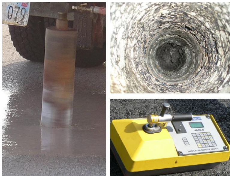
Figure 1. Illustrations of core sample test and nuclear test methods: (a) Coring; (b) coring hole, and; (c) nuclear gauge
