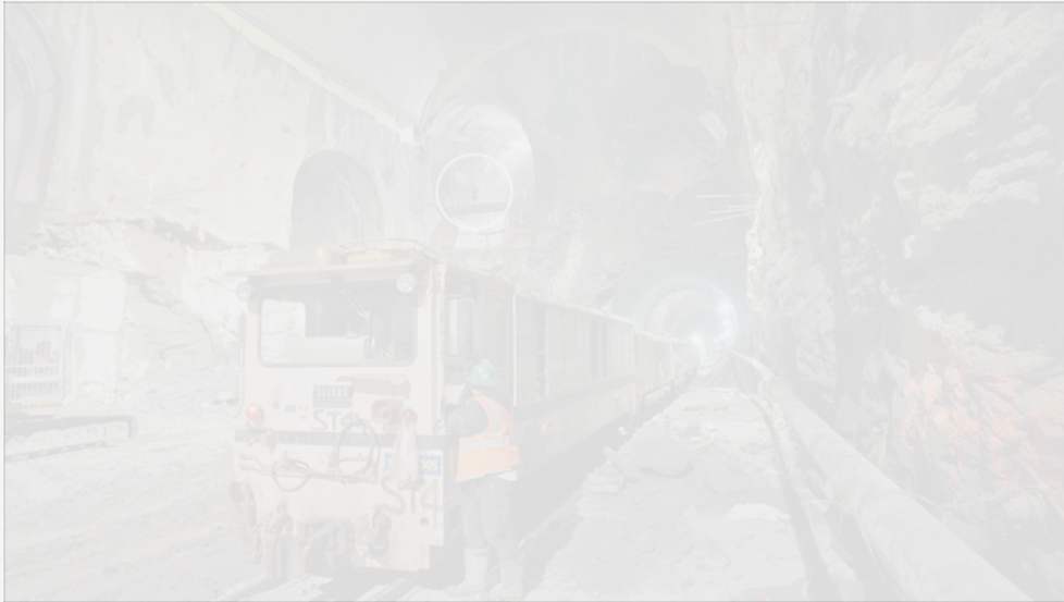
The Second Avenue Subway offers one alternative to digging into city streets to install the tubes. Image via the MTA .
