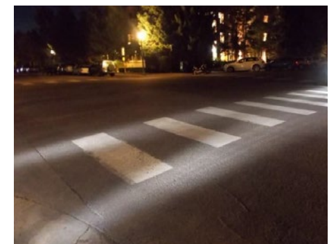
LED Bollard Luminaires Tested in Colorado
