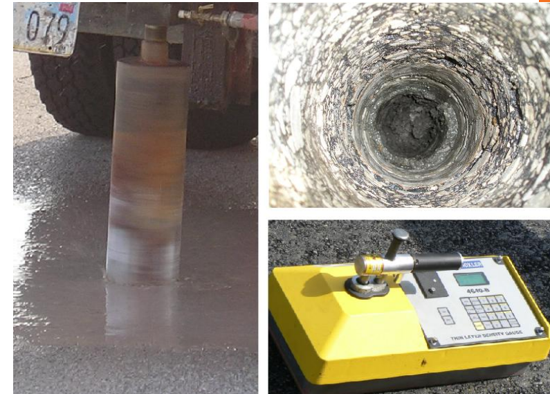
Illustrations of Core Sample Test and Nuclear Test Methods: (a) Coring; (b) Coring hole, and; (c) Nuclear gauge
